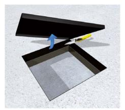
5 | Cut out opening After the screed has hardened remove the overlapping lid and sidewalls neatly. Side walls must be maintained.
