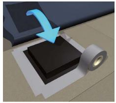
3 | Mounting of foil Fix shuttering units to the floor with adhesive tape, cut out foil and overlap.
